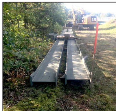
I-beams ready to go!
