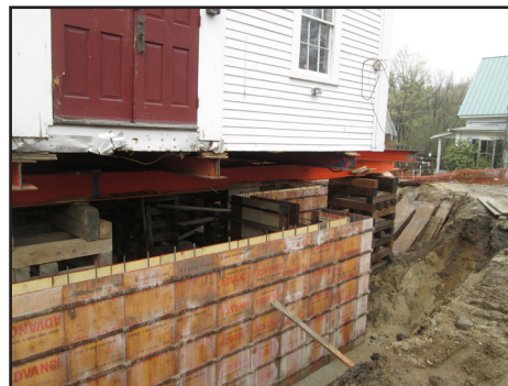
Foundation forms under the front of the building.
