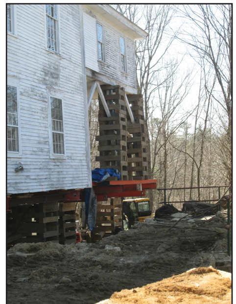
Extensive cribbing supports the second floor extension.
