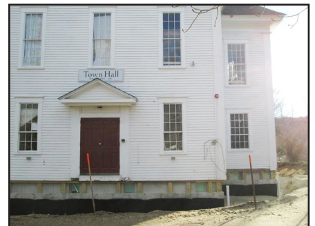
Left: Town Hall on new foundation from the parking lot. Right: Front entrance of Town Hall after it was lowered onto the foundation.
