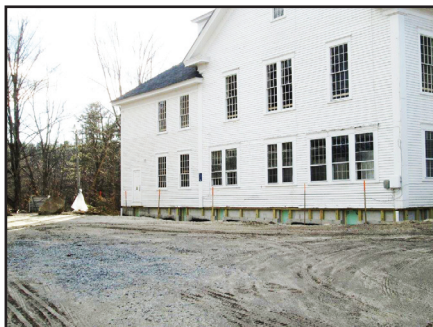
Left: Town Hall on new foundation from the parking lot. Right: Front entrance of Town Hall after it was lowered onto the foundation.
