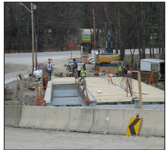
Bridge takes shape
