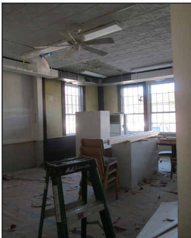
Planning Board office wall removed
