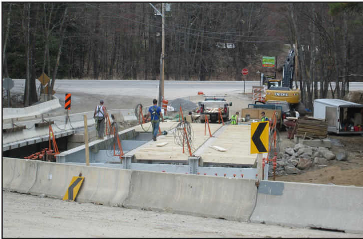
Preparing for the deck
