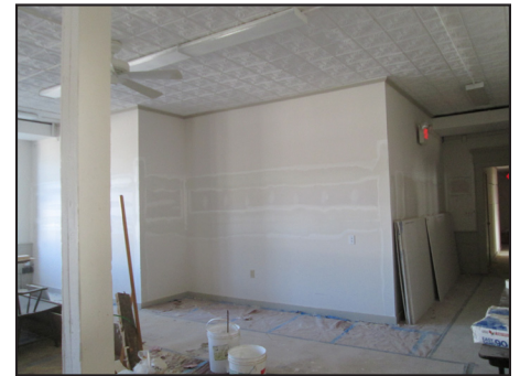
Patched and ready to paint
