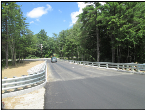
Breezy Hill Bridge Route 103 end open for traffic
