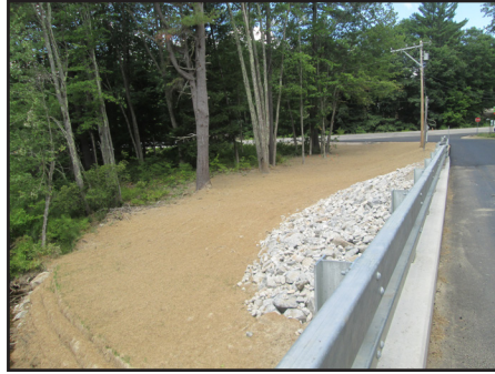
Temporary bridge on Breezy Hill Road as been removed
