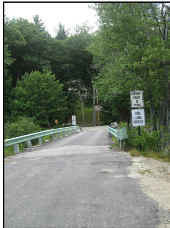
Pond Bridge heading toward Route 103
