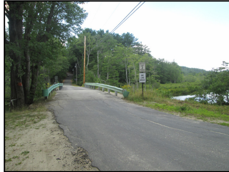
Pond Bridge towards Route 114
