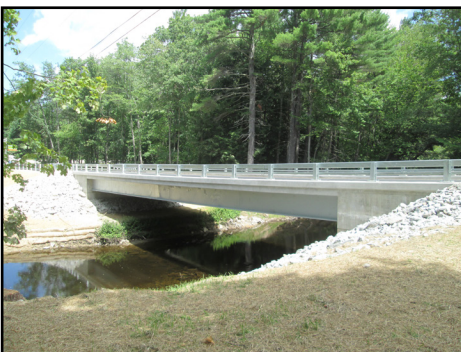
Breezy Hill Bridge from the river
