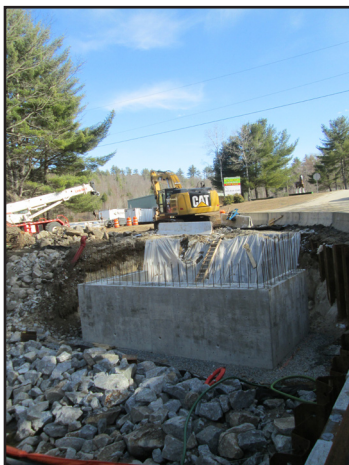
Abutment being formed for the replacement bridge on Breezy Hill Road
