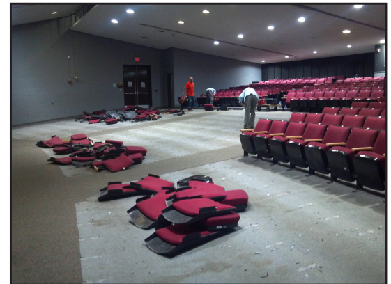
Old seats being removed
