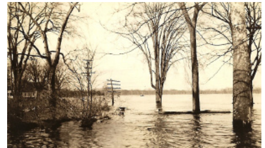
Telephone communication disrupted by flooding.
