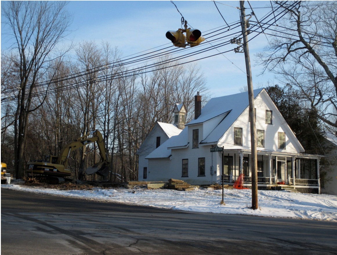
Corner of Old Warner Road and Route 114, post demolition
