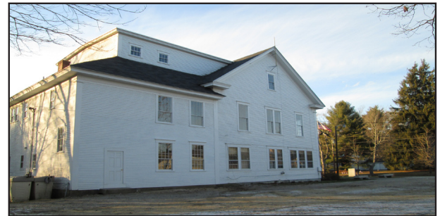
Note new white membrane roof on flat portion of the building.
