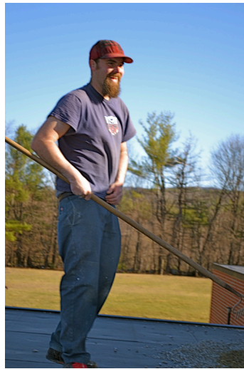
Travis spreads peastone on the roof of KRES
