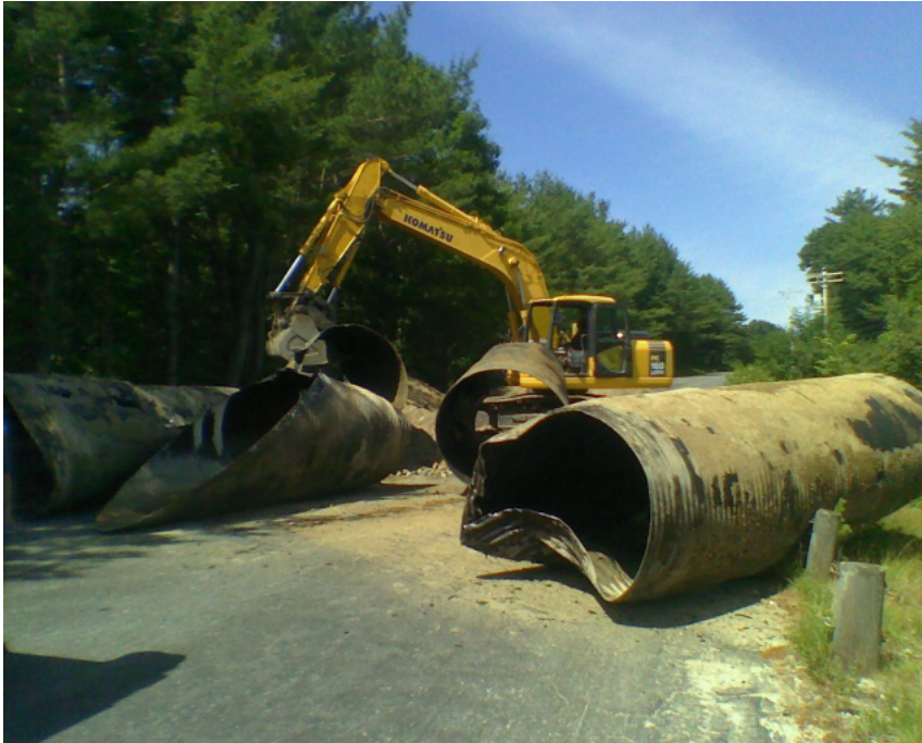
Replacing a culvert on Old Warner Road
