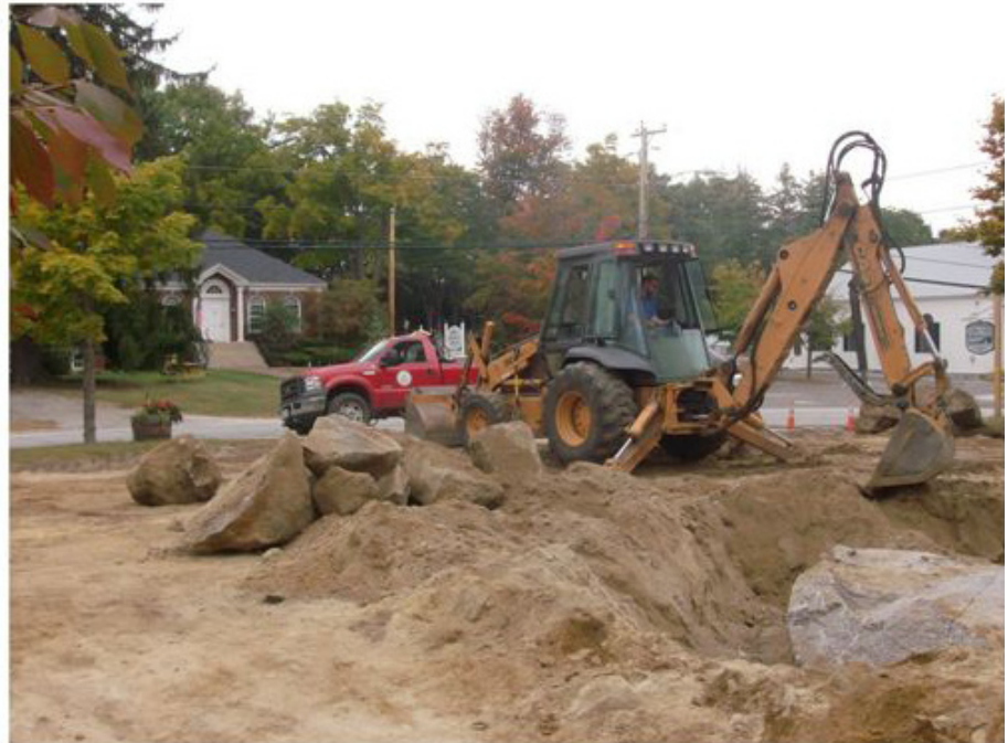
The town hall parking lot undergoing repaving
