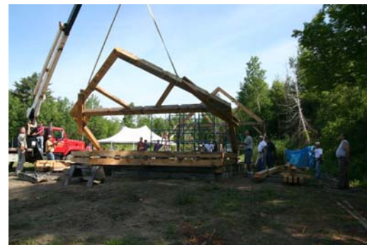
with some help from machinery
