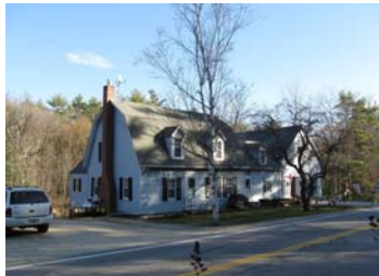
SUTTON - In home business setting for this immaculate 1840's gambrel with new kitchen, granite counters, maple cabinets, large LR, family room, 2.9 acres, many new updates. Existing successful gift shop is also available for additional price. Lots of traffic & parking. Call for details. $295,000.00
