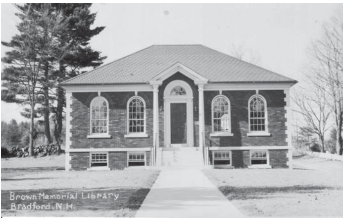
Brown Memorial Library, exterior view 1932
