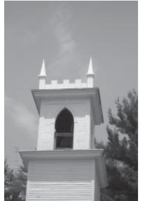
The Bradford Center Meetinghouse has undergone extensive repairs, including structural repairs to the roof and steeple, both of which have suffered water damage for years. Bruss Brothers Construction has replaced the rotted areas with man-made material that will last for years to come. Above are two finials, one of which has totally disintegrated. Right: the replaced finials adorn the repaired steeple.
