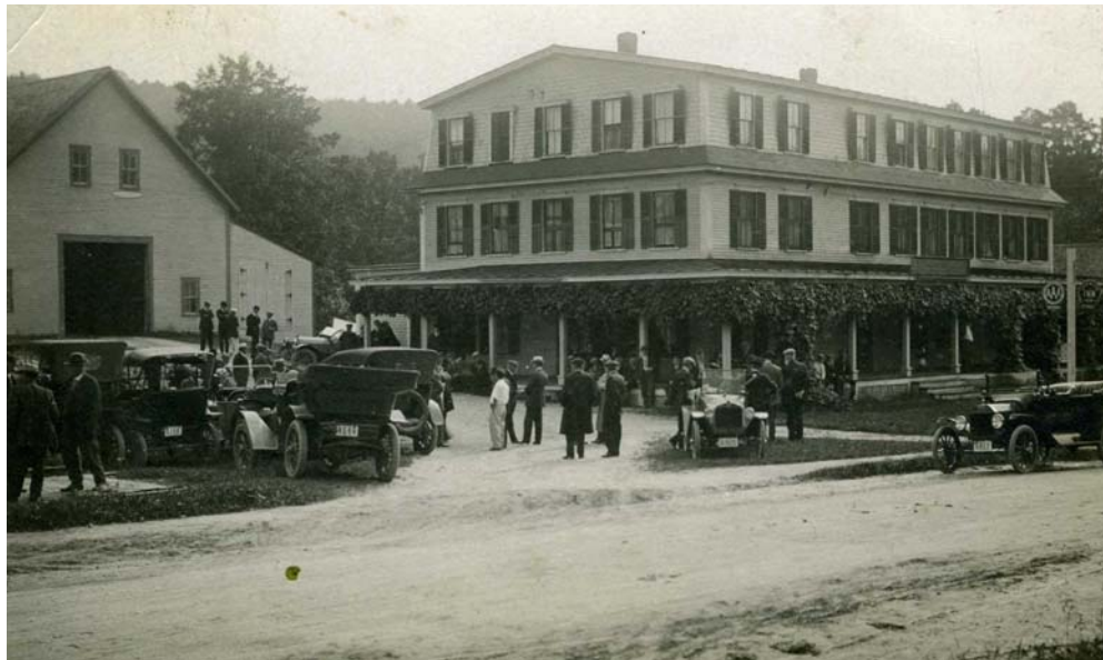
April, 1898, The "New Bradford Hotel" has been constructed on the site of the old one, and the plumbers are at work. The upper story contains 26 sleeping rooms, the heating apparatus is the latest from C.H. Marshall, and the current is furnished by the Bradford Power and Light Co. A good all around pastry and meat cook from Boston has been engaged and all the arrangements of the hotel will be of first class order.
