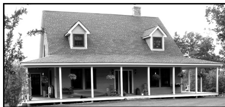
SUTTON: Custom built home w/ eat-in kit, den could be converted to dining rm; hwdw flrs, in living rm, upstairs; carpeting, marmoleum in baths and inlaid in kitchen, pantry storage, farmer's porch-3 sides. Terrace off bsmnt. Lg yard, outbldg, Fplc & 9' ceilings. Horses poss. $389,000
