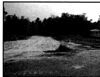
A 21-lot subdivision proposal is pending for this Fairgrounds Road site (left). A home on West Meadow Road is near completion (below left) while work begins on a foundation for a home in a Cressy Road subdivision (below right.)
