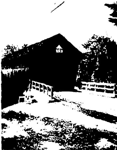
The first phase of the Bement Bridge repairs involved installing wood-clad steel approach rails designed to complement the historic nature of the bridge.
