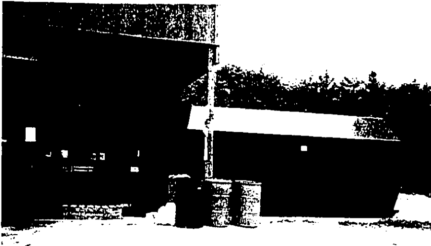
Compactor and closed box installed at Transfer Station in time for busy July 4th weekend. Except for the color, the equipment looks similar to what has always eaten your trash, but this one is our own! (or will be at the end of a three-year lease.) The monthly cost is less than the previous rental and, when the purchase is final, the savings will total $575 per month. A good investment. Ken Anderson, Transfer Station Manager, commented that "It will be good to have our own equipment."
